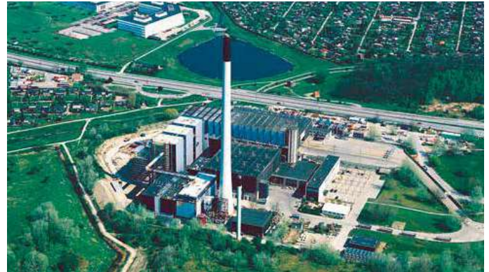
Vestforbrænding - Waste-to-Energy Plant in Copenhagen
