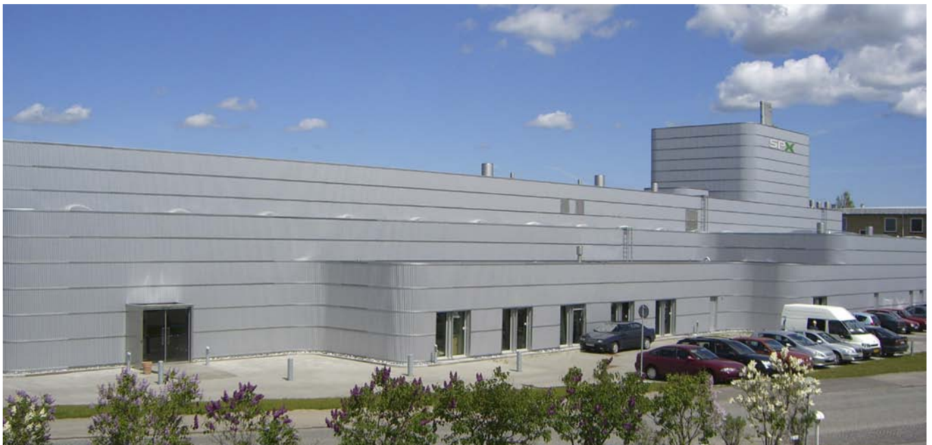
SPX innovation center in Soeborg, Denmark
